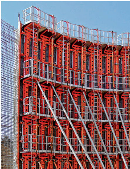
With the appropriate platforms, guardrails and access ladders, safe working and concreting scaffolds can be realized.
