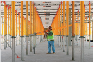
Slab Formwork
