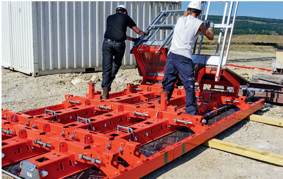
Assembly of the accessories is carried out on the horizontally-positioned panel. During the moving procedure, everything remains mounted in position.
