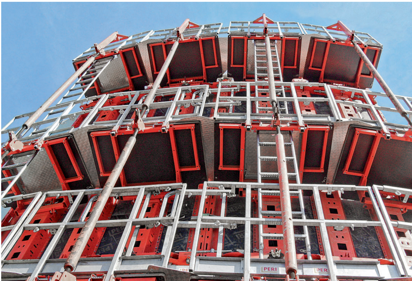
Assembly of the accessories is carried out on the horizontally-positioned panel. During the moving procedure, everything remains mounted in position.
