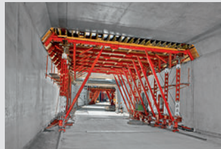
Tunnel Formwork
