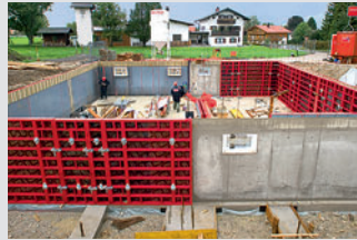
Wall Formwork
